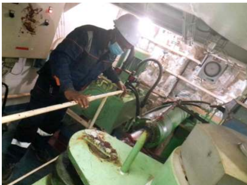
GUINEA PSCO INSPECTING STEERING GEAR HYDRAULIC SYSTEM
