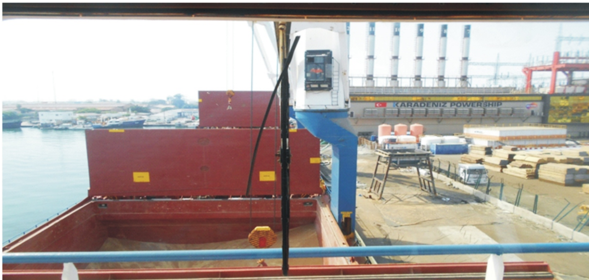
Bulk Carrier hatch cover inspection
