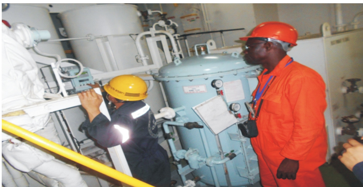
Inspecting oily water separator
