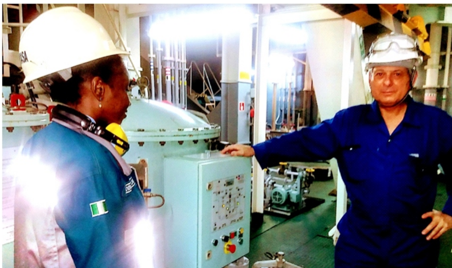
Inspection of Oily water separation controls
