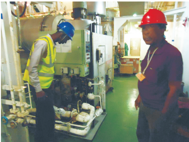
PSC Inspection on Incinerator, The Gambia.
