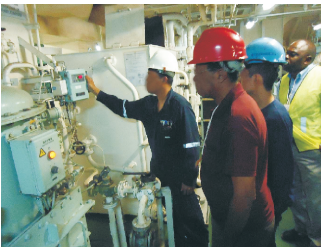
PSC inspection on oily water Separator, The Gambia.
