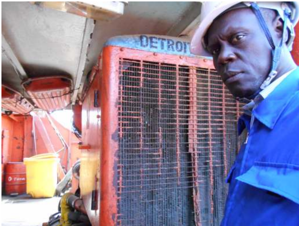
Senegal PSCO Inspecting a Rusted and Damaged Engine Cooling System Radiator Grid
