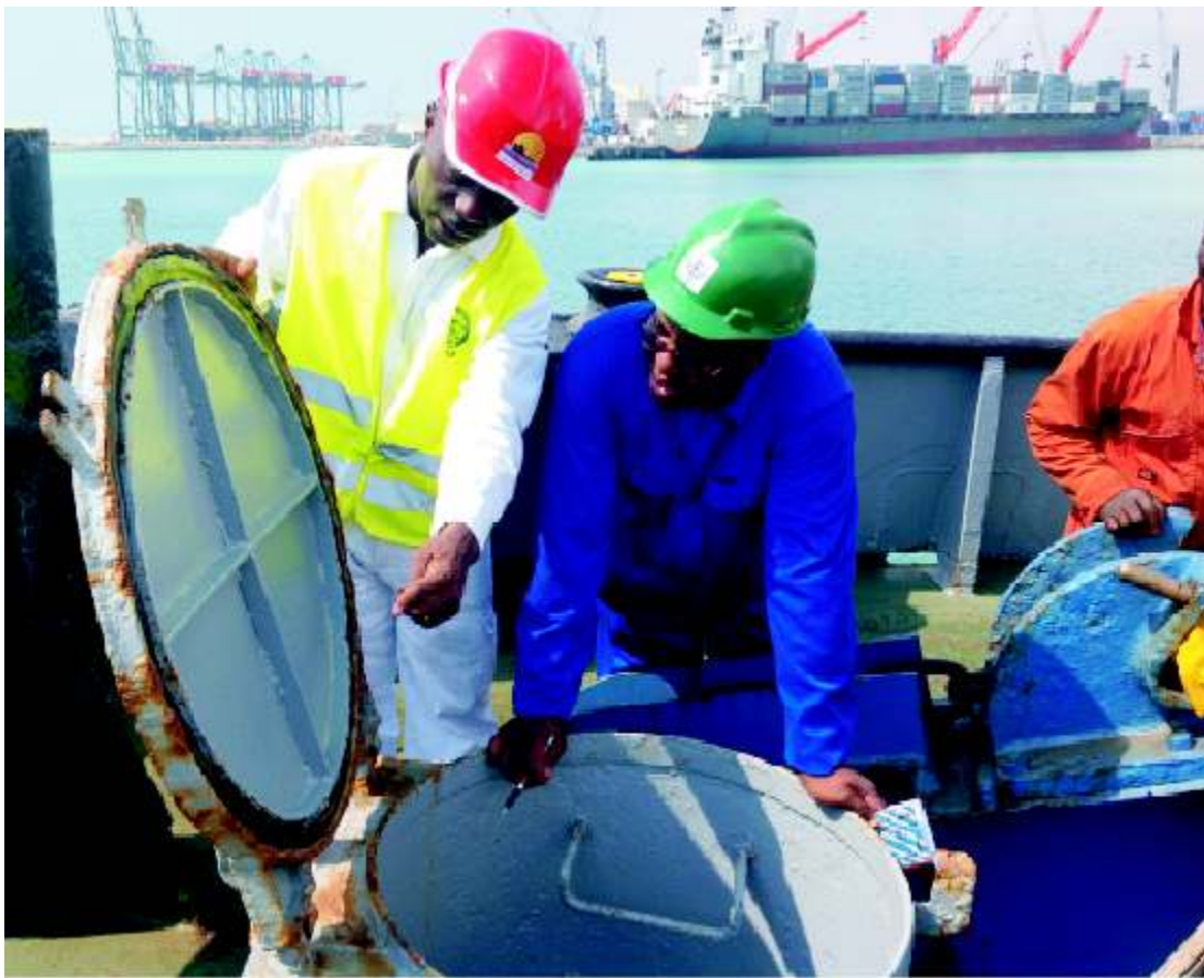
Ghana PSCOs inspecting the rusted and wasted water tight door on Escape Hatch
