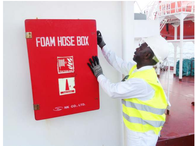
Ghana PSCO Inspecting Fire Water Hose Box
