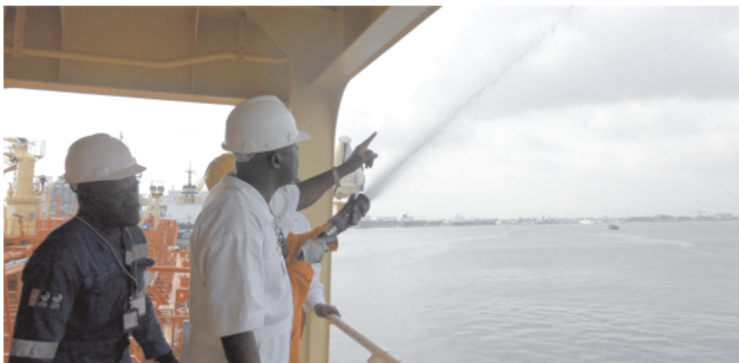
Fire fighting water jet test
