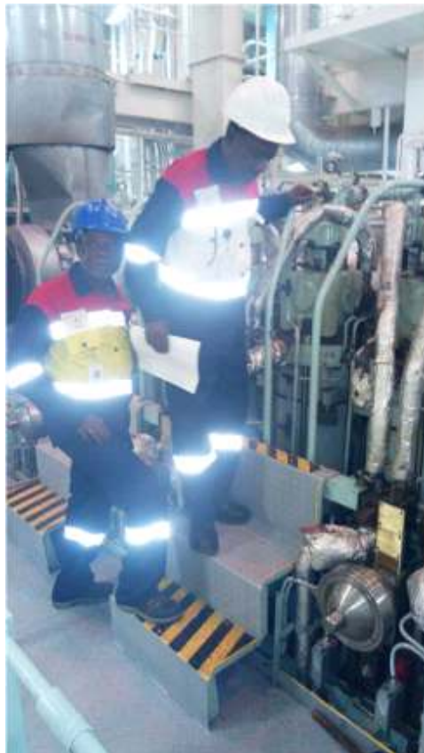
PSCOs on top of main propulsion engine
