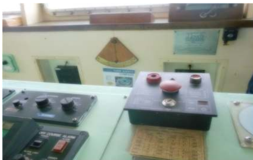
On the Bridge Clinometer, Alarm panel, Emergency stop button
