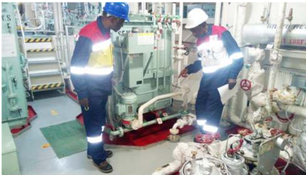
PSCOs inspecting Sewage plant lines
