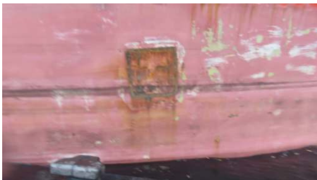
Corroded Repaired Ship Hull
