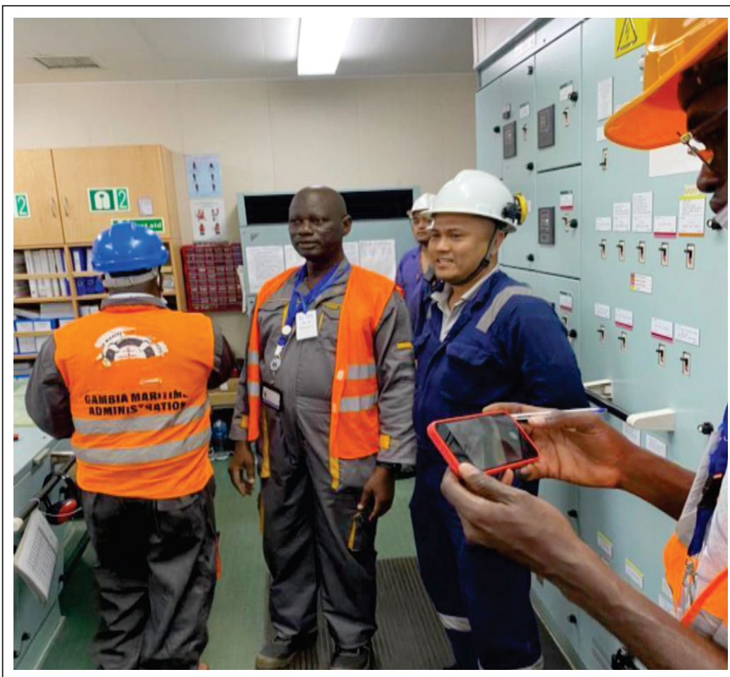
PSCOS inspecting Engine Control Room
