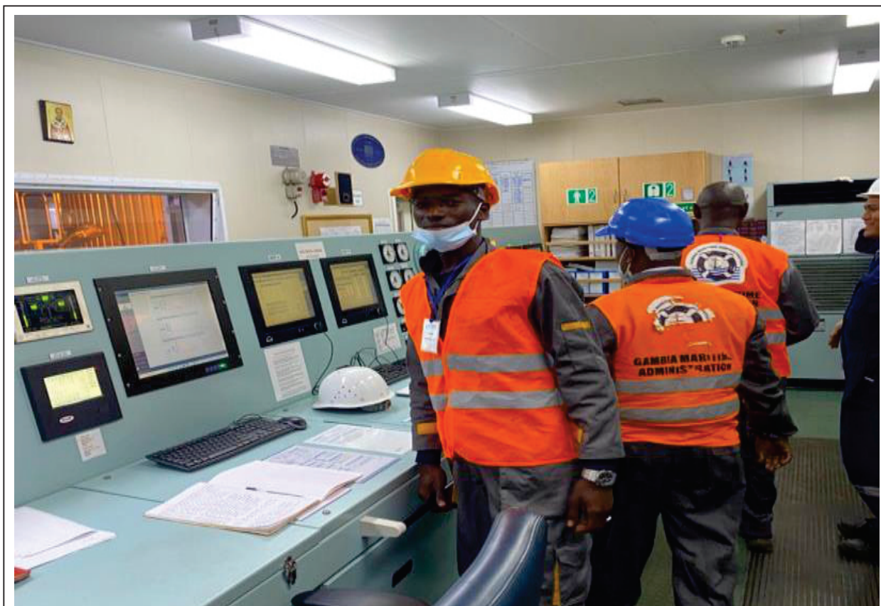
PSCOS Inspecting the Engine Control Room
