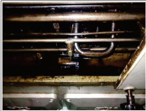
auxiliaries' engines cylinders leaking oil
